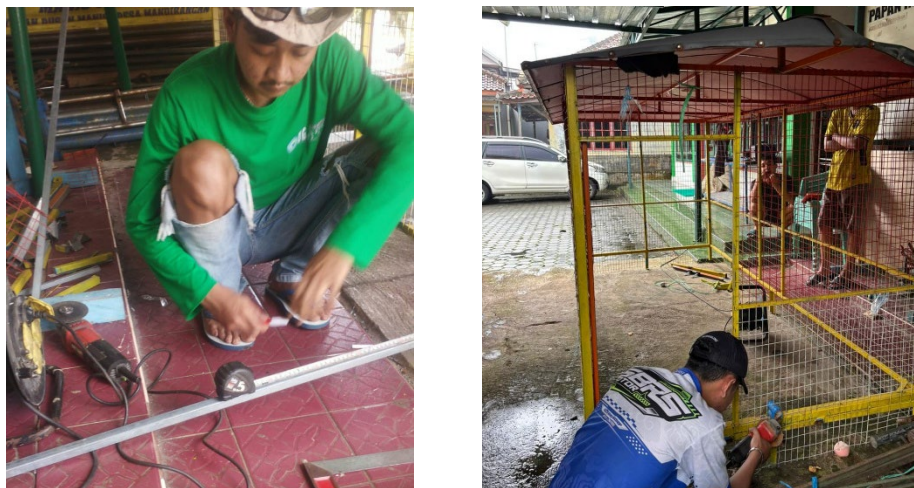
Figure 2. Waste bin construction process
