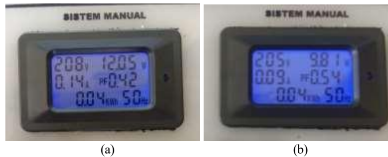
Figure 6 Measurement Results Before Power Factor Repair (a) TL Lamp: (b) Fan
