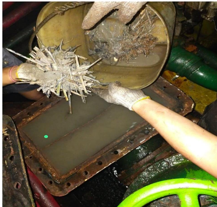
Figure 14: Dirt Accumulating in the Master Machine Strainer. Source: Personal documentation
