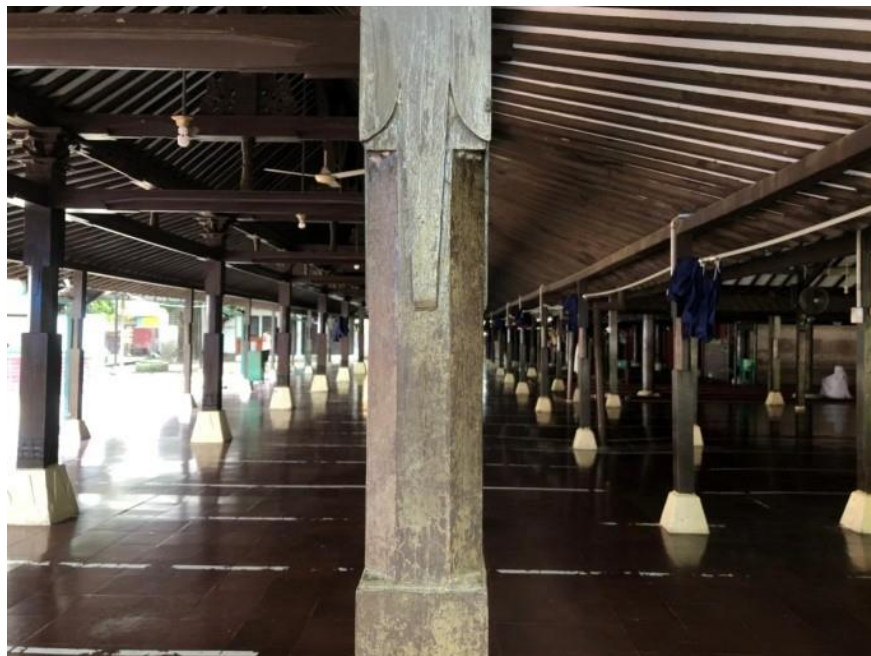
Picture The position of the poles supporting each other in the Sang Cipta Rasa Mosque Sumber foto An Nuur Khairune Nisa
